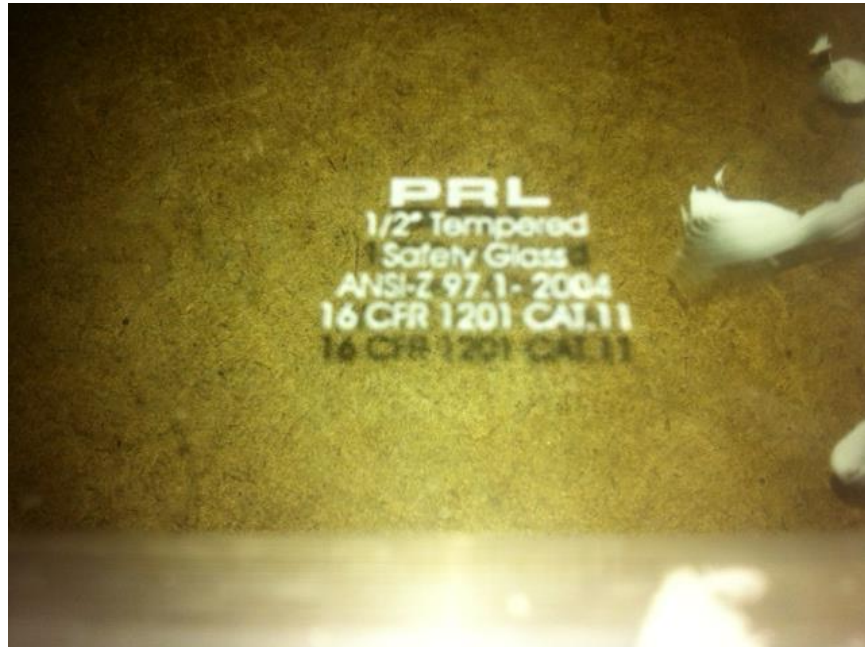
Photo No. 1 Typical identification of glass panel
